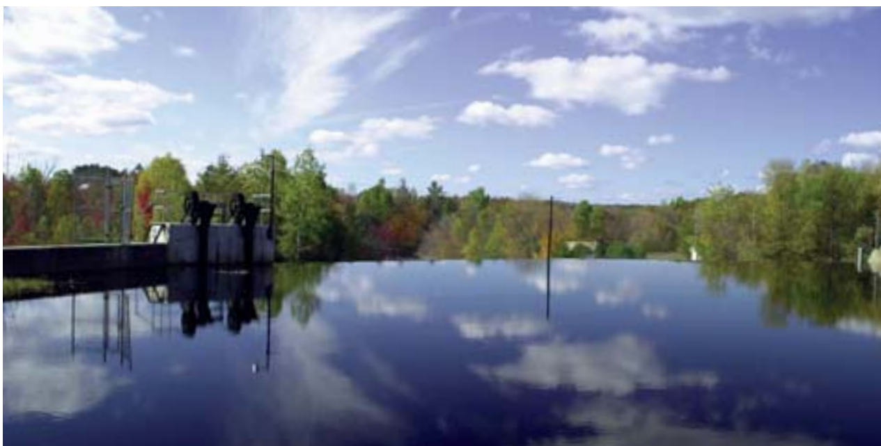
FortisUS Energy owns and operates 4 hydroelectric generating stations in upper New York State with a combined capacity of 23 MW.
