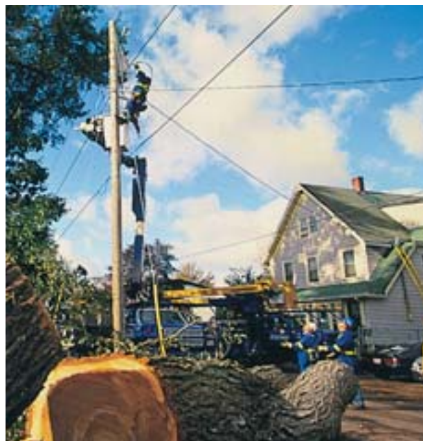
Employees work to restore power to customers impacted by Hurricane Juan.
