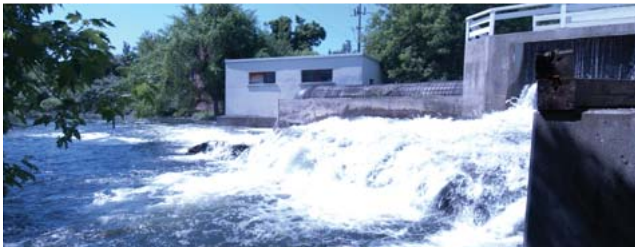
Washburn hydroelectric generating station, Rideau Canal.
