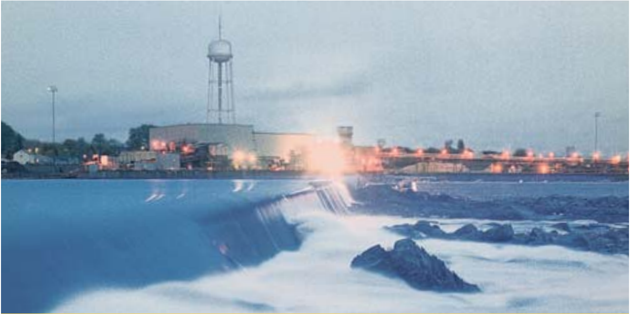
The Exploits Partnership project is a redevelopment of Abitibi-Consolidated's hydroelectric facilities in central Newfoundland.
